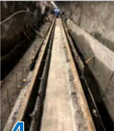
Remove shutters. T-Track installation complete
