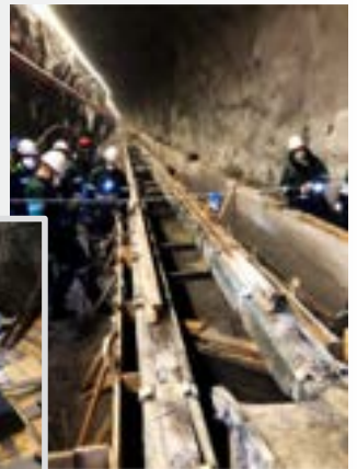
Place modules along centre line, install rail and fasten to module, lift and align track to specification and install shutters. Place concrete (filler grout) under modules.
