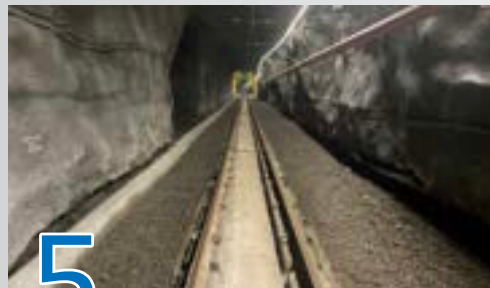
Backfill side of track for walk ways
