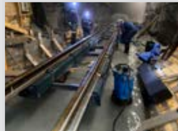
Place modules along centre line, install rail and fasten to module, lift and align track to specification and install shutters. Place concrete (filler grout) under modules.
