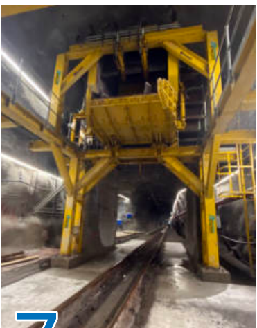
4 Remove shutters. T-Track installation complete
